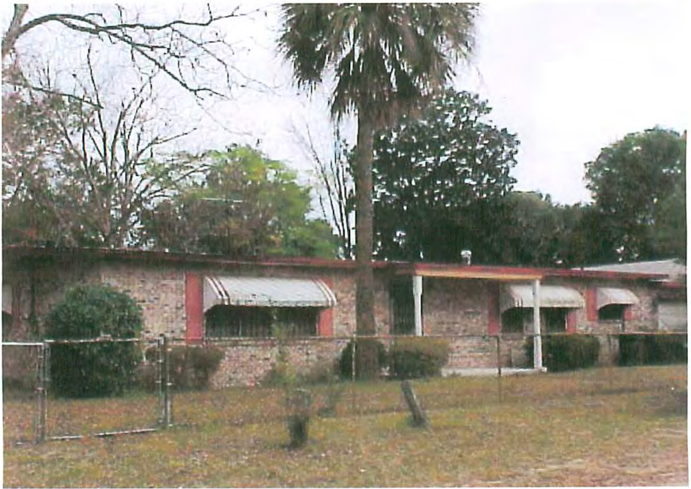
Sanitary Sewer Connection 3218 North Tarragona
