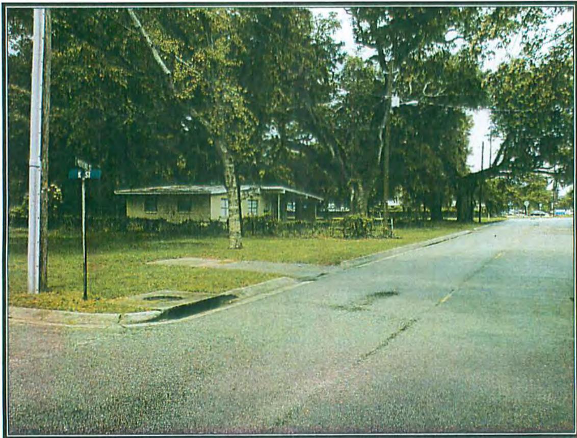
View along Moreno Street (Subject on left)
